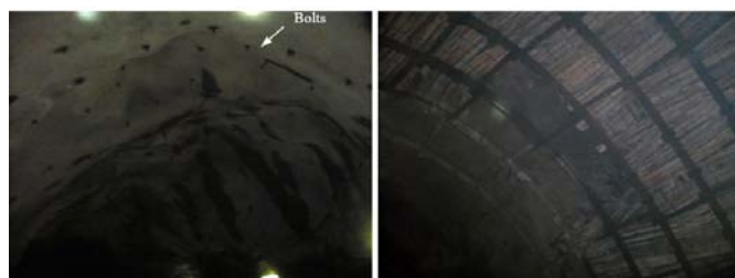
Fig. 2 Places with reinforced support in the ramp
