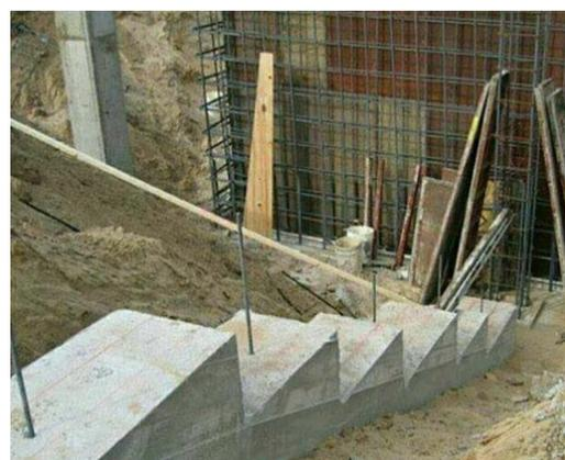
Fig. 1 Execution of stepped foundation in sloping lands
